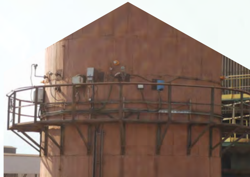
Part of the installed equipment for Continuous Emission Monitoring
