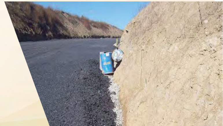
Using slag as a road base
