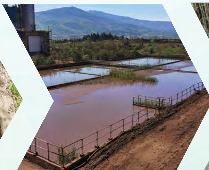
Return of the water to sediment in the Thickener and Sedimentation Pools
